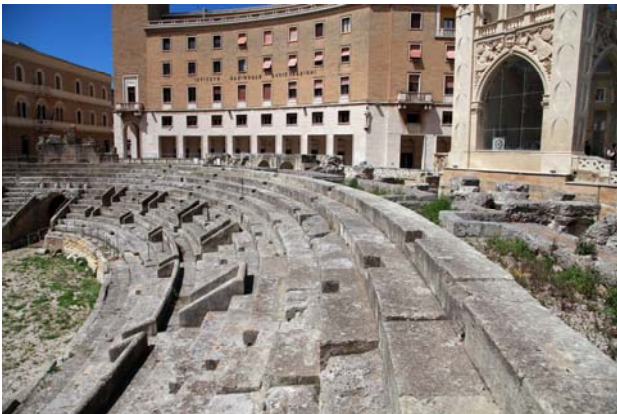
Fig. 5. The actual cavea with the remains of vomitoria , is clear the impossibility of praecinctio .
